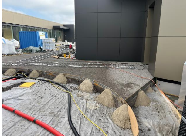
Profile installation without ground anchor in concrete foundation (point foundation)
