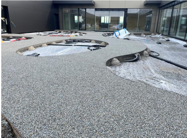
Profile installation without ground anchor in concrete foundation (point foundation)
