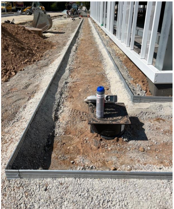
Profile installation without ground anchor in concrete foundation (strip foundation)
