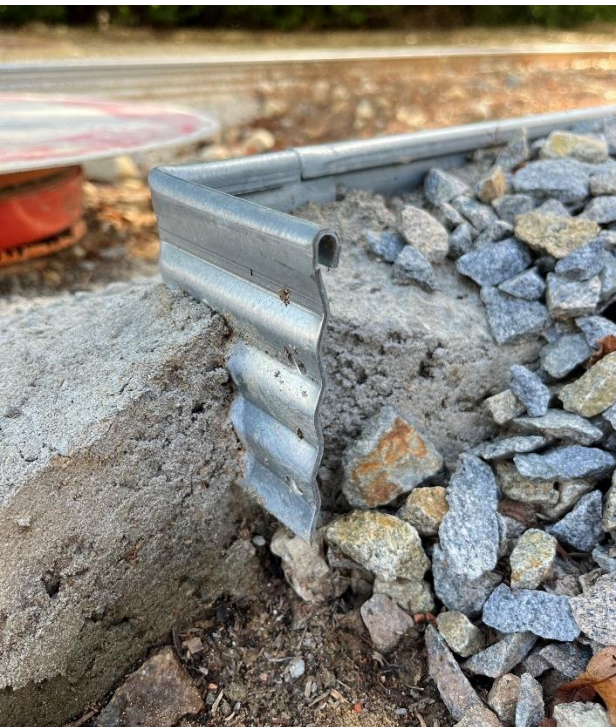
Profile installation without ground anchor in concrete foundation (strip foundation)
