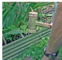
► Use a plastic hammer for inserting the profiles. Do not directly hit the profile with a metal hammer as it might get damaged and possibly will corrode due to flash rust. Use the edge knocker for protection.
