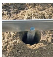
► Ground fixations are used in case the corrugated profile does not provide sufficient stability in the ground. Installation in gravel, crushed stones, tightly curved edgings or slopes are typical applications to use ground fixations.
