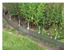
► First the profiles are screwed together. Then prefix the profiles in the desired shape (straight or curved). Use the positioning bars which have a guide pin to anchor the profiles. The positioning bars are removed after installation. You can reuse them for your next project.
