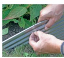
► In case of natural soil it is advisable to pre-cut the ground with a shovel alongside the profiles. Remove rubble, stones and roots before you start installation. If the ground is hard or dried-out, it is better to water first.
