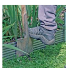
► The installation of the profiles depends on the application and soil conditions. Either the profiles are inserted directly into the ground or the ground is pre-cut with a shovel. The edgings of roads and paths are set in concrete foundations. Check before installation, whether in the ground are tubes or pipes.
