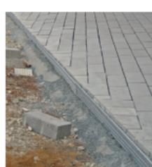
► Alternatively to the use of ground fixations, the profiles can be stabilized with in concrete foundations when being installed in gravel or grit.
